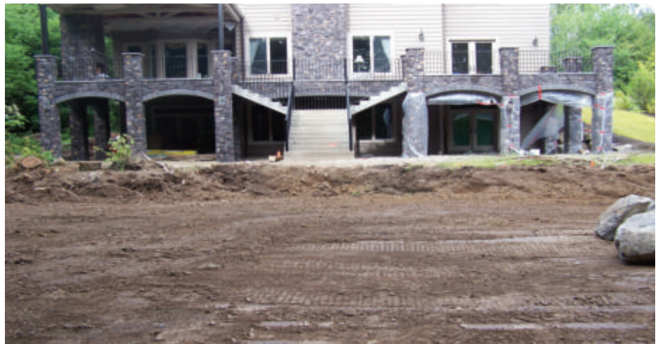
The site before excavation
